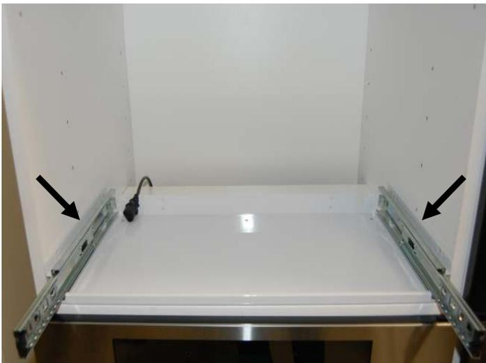
1) Put the base on the case, left and right side in contact by the panel
