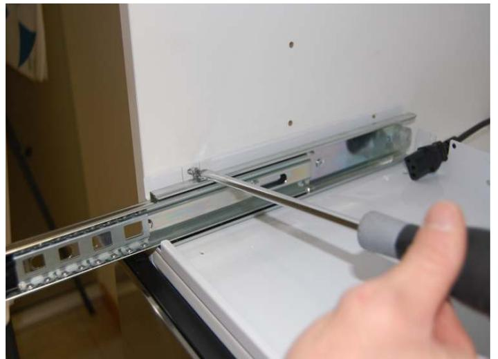
3) Screw the base to the sides (using the x4 screws provided)
