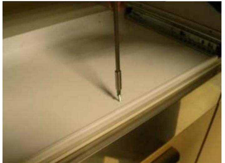
2) Screw the base on the case (using the x6 screws provided)
